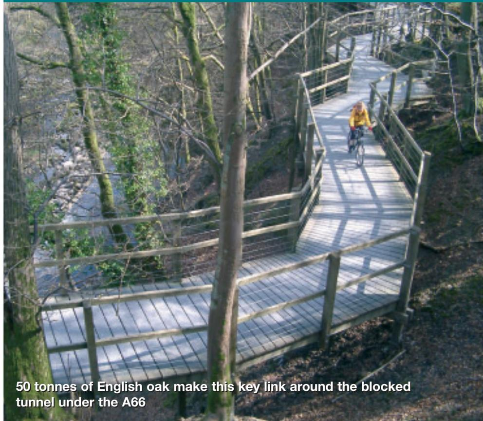
**50 tonnes of English oak make this key link around the blocked tunnel under the A66**
